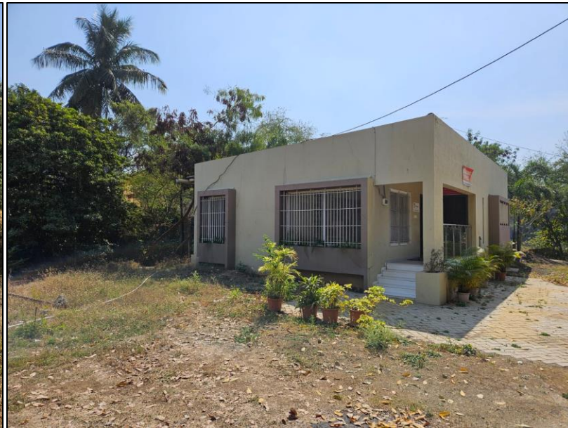
C Wing : Site office
