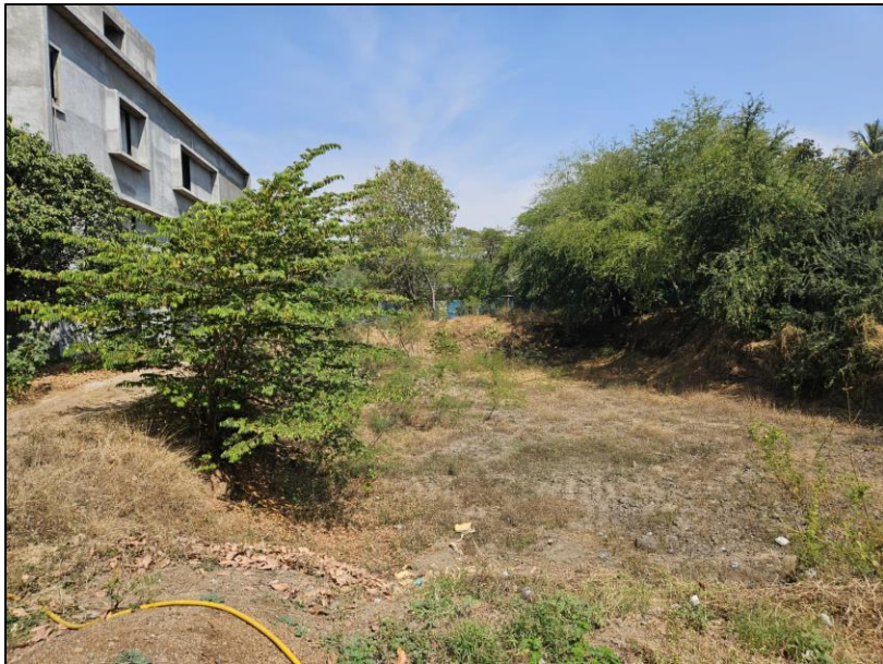
C Wing : Part excavation done
